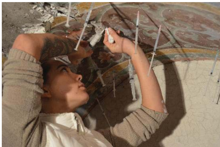
Injection of Acrylem and Ledan Tb1 into process one of the arches.
