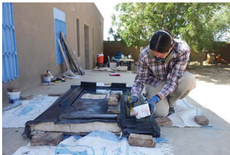
Application of carbon fibre and epoxy resin during realisation of the support.
